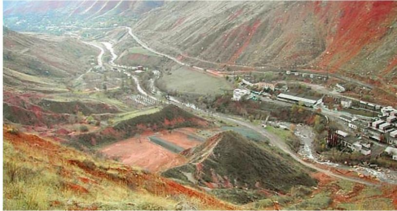
**Figure 5.** Valley of Mailuu-Suu, showing the former ISOLIT processing plant on the right and the relocated tailings dump no. 3 on the left side/center.
